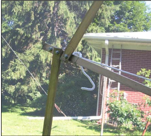
Figure 4. An outside rim is formed from 3.5' length of ½" x ½" modeling strips
