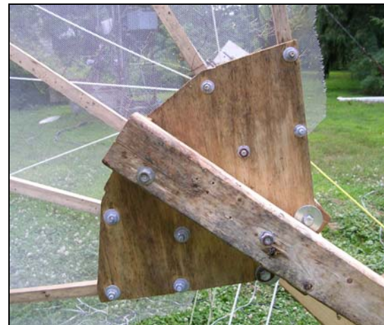
Figure 3. The struts are attached to a square plywood center with two bolts
