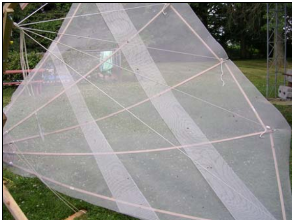
Figure 9. Aluminum screening is tie to the struts using wire
