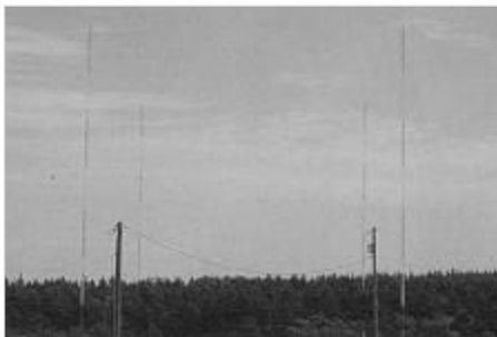
Antény VY2ZMM - 4 square pro 160m (op. K1ZM, K2WI, WW2Y)
